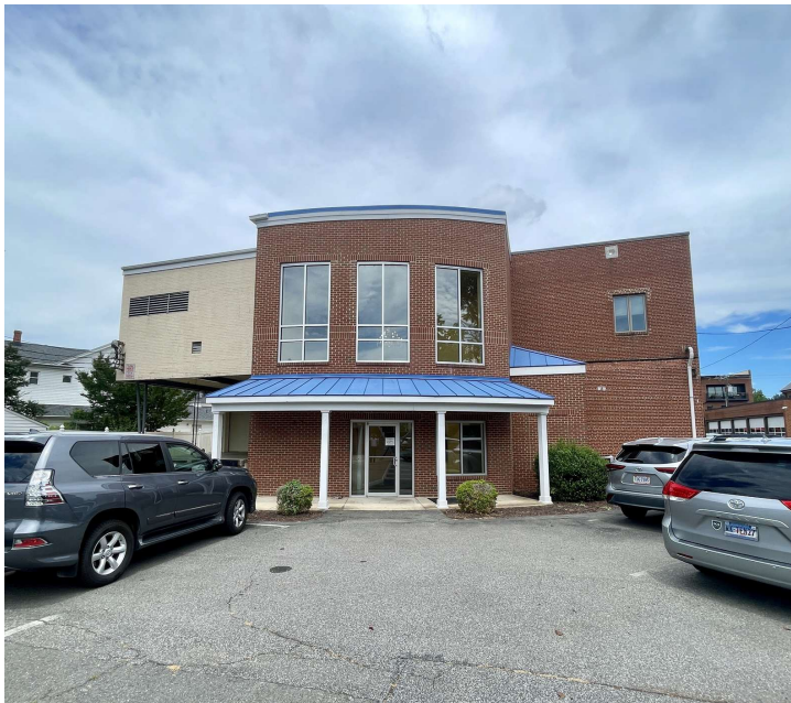
Existing Rear Entry Door, Pre-Renovation
