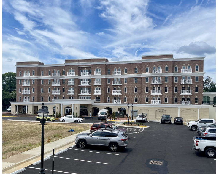
The Publisher Hotel, a Marriott Tribute Portfolio Hotel featuring 98 rooms and Five Chophouse, a brand new on-site full-service restaurant and bar
