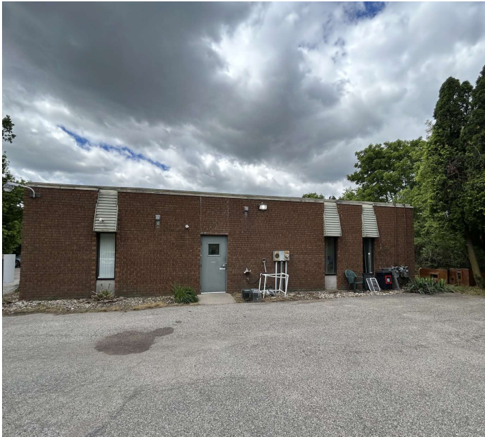
Back of Building
