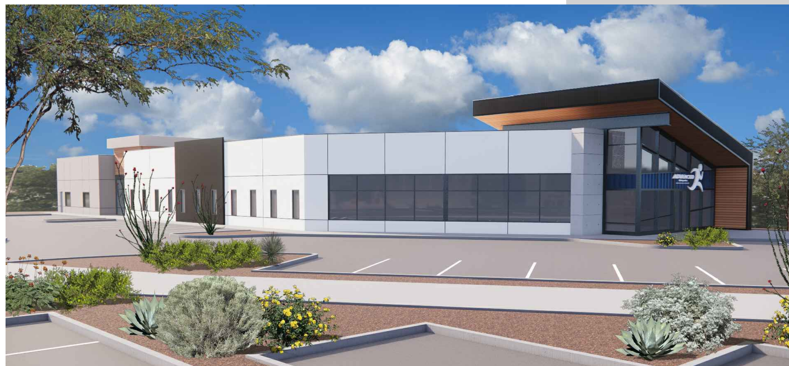
View of M.O.B. from parking
