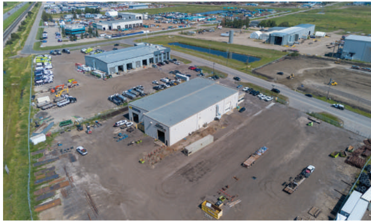
South side of shop
