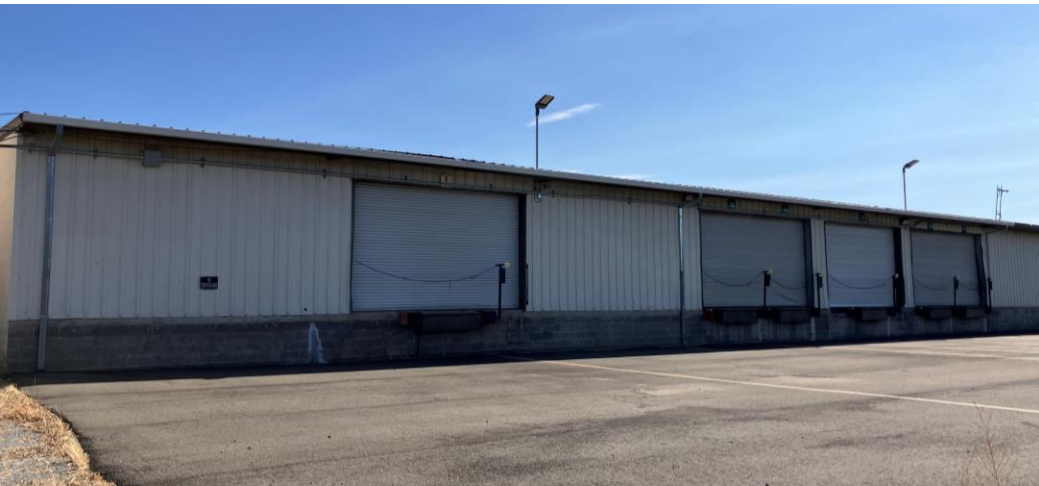
Back Loading Docks
