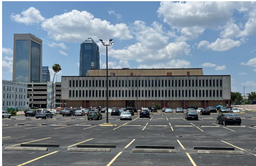
West view of the Fuller Warren Building
