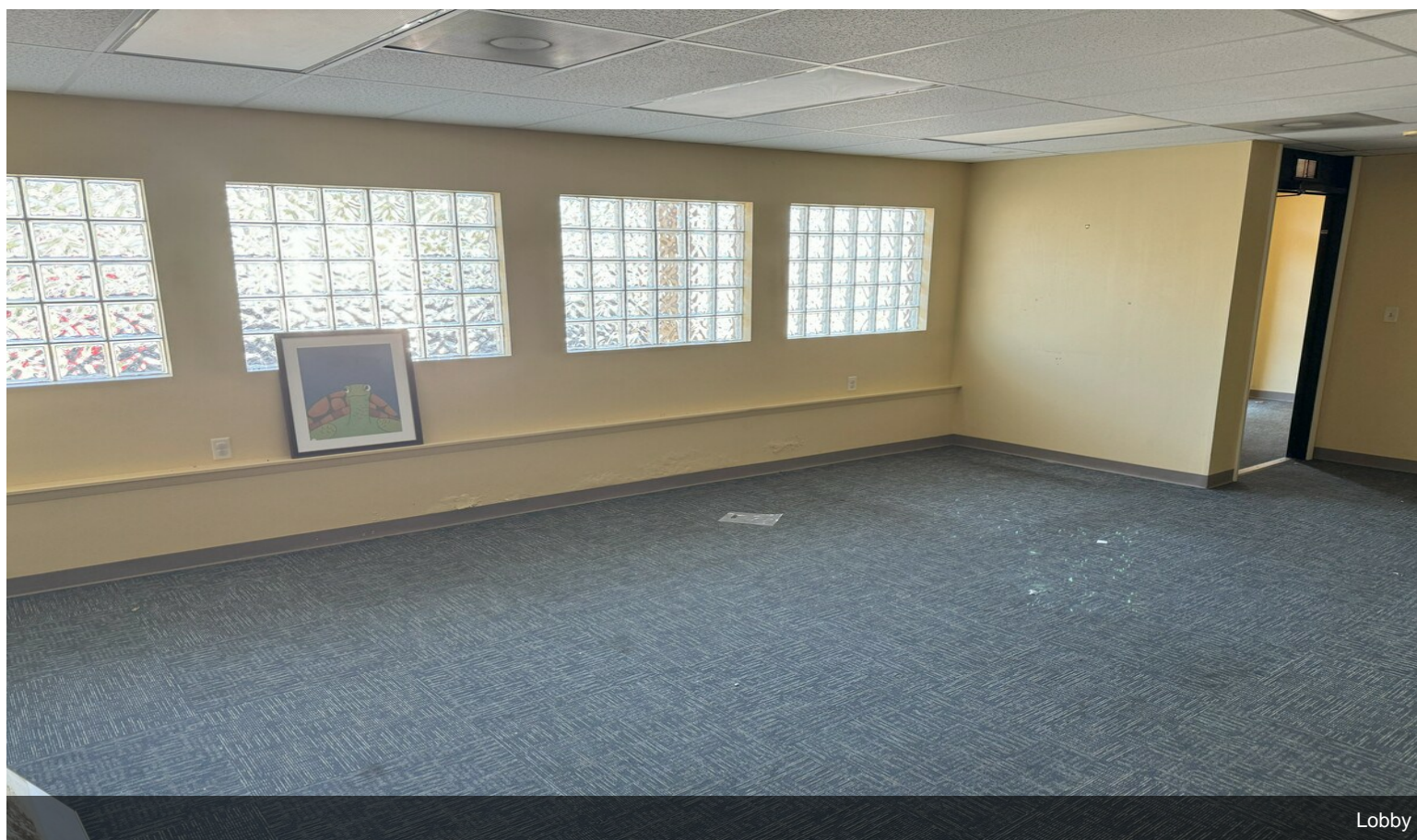
Lobby facing Front Door
