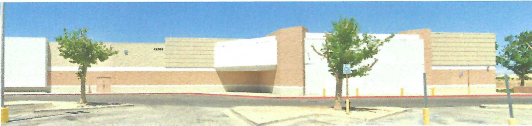
Existing Condition - East
