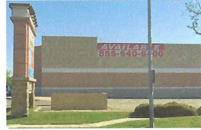
Existing Condition - North
