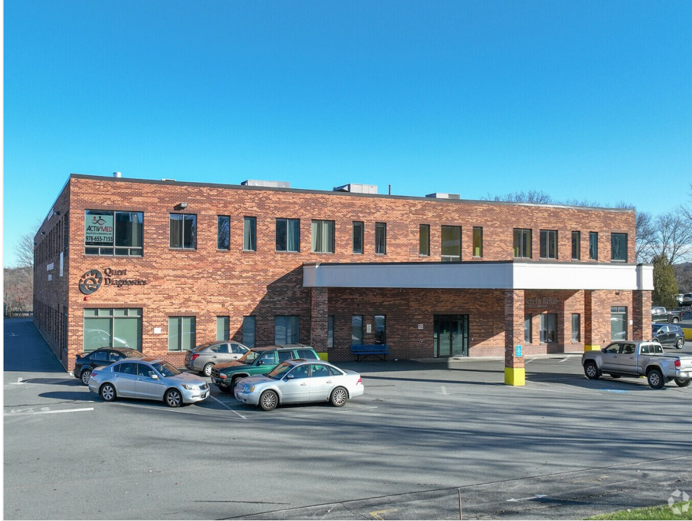
Alternate Angle of Front of Building
