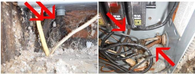
SAFETY ALERT. The wiring is a combination of the original cloth insulated copper wiring and the plastic insulated copper wiring. The cloth covered wiring is old and may continue to function unless it is disturbed or overloaded.
