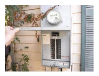
MAIN PANEL AMPERAGE Service Amperage - 200 Amps.
