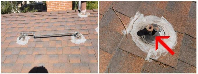
**NEEDS ATTENTION.** There are penetrations in the roof that are damaged and may allow moisture to enter the bldg.
