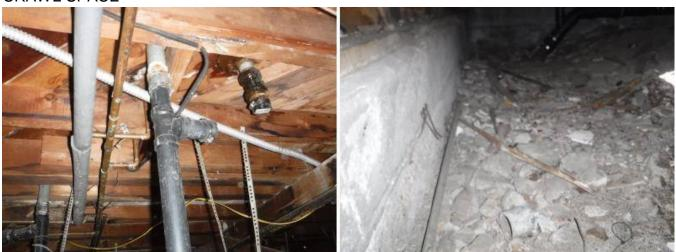
**NEEDS ATTENTION.** The crawl space has debris in it, it is advisable to have this removed and the area cleaned up. Wood especially should be removed to help prevent future infestations.
