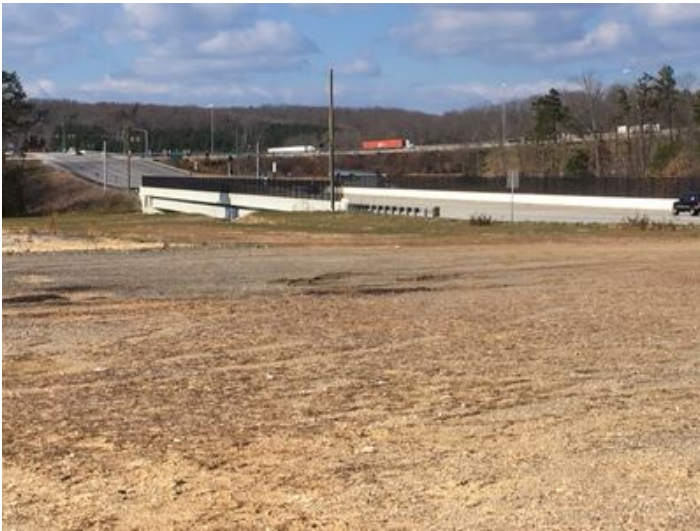
Level, Graded, Compacted Pad Site
