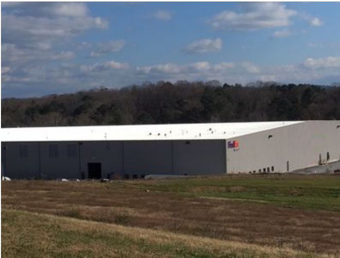
Newly installed FedEx Distribution Center on the Interchange
