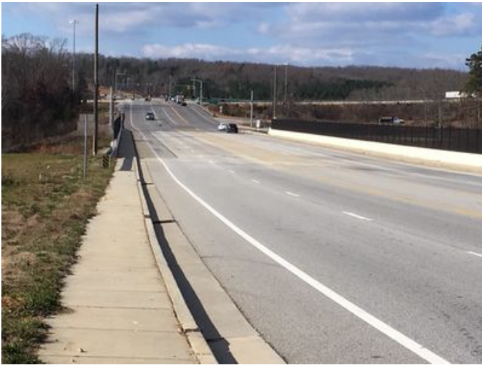
Property is located at the South East Quadrant of Exit 9, Volkswagen / Apison Pike
