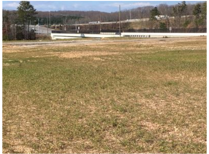
New TDOT Bridge and Road Improvement Project
