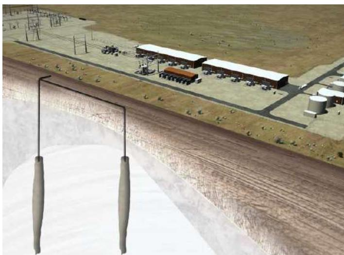
(9) Chevron and Mitsubishi Power's ACES Delta project near Delta, Utah will be one of the world's largest green hydrogen storage hub. Using 220 MW of electrolysis, it will produce 100 metric tons of hydrogen daily, stored in vast underground salt caverns holding 300+ GWh of dispatchable energy. Linked to the Intermountain Power Project, it enters commercial operations in 2025 to supply utilities, industry, and transportation.
