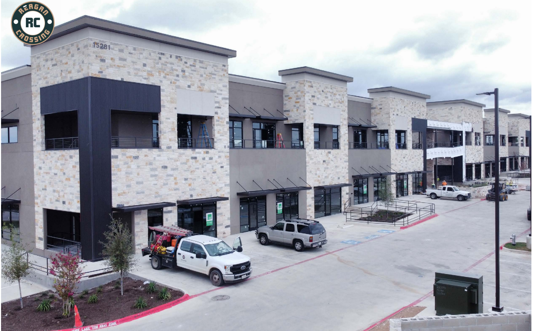
CONSTRUCTION PROGRESSION AS OF SEP 2024
