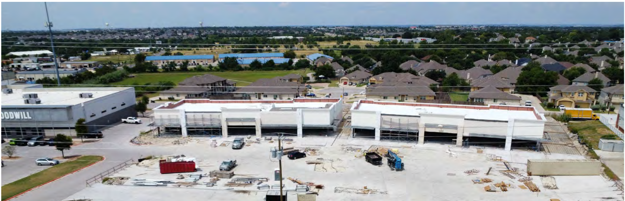
Construction Progression August 2025
