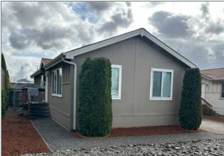
UNIT #6 NORTH SIDE
