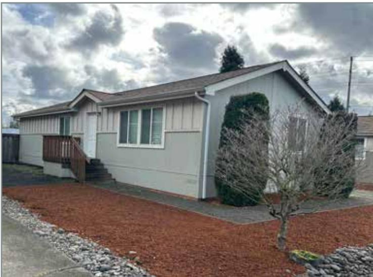
UNIT #4 NORTH SIDE
