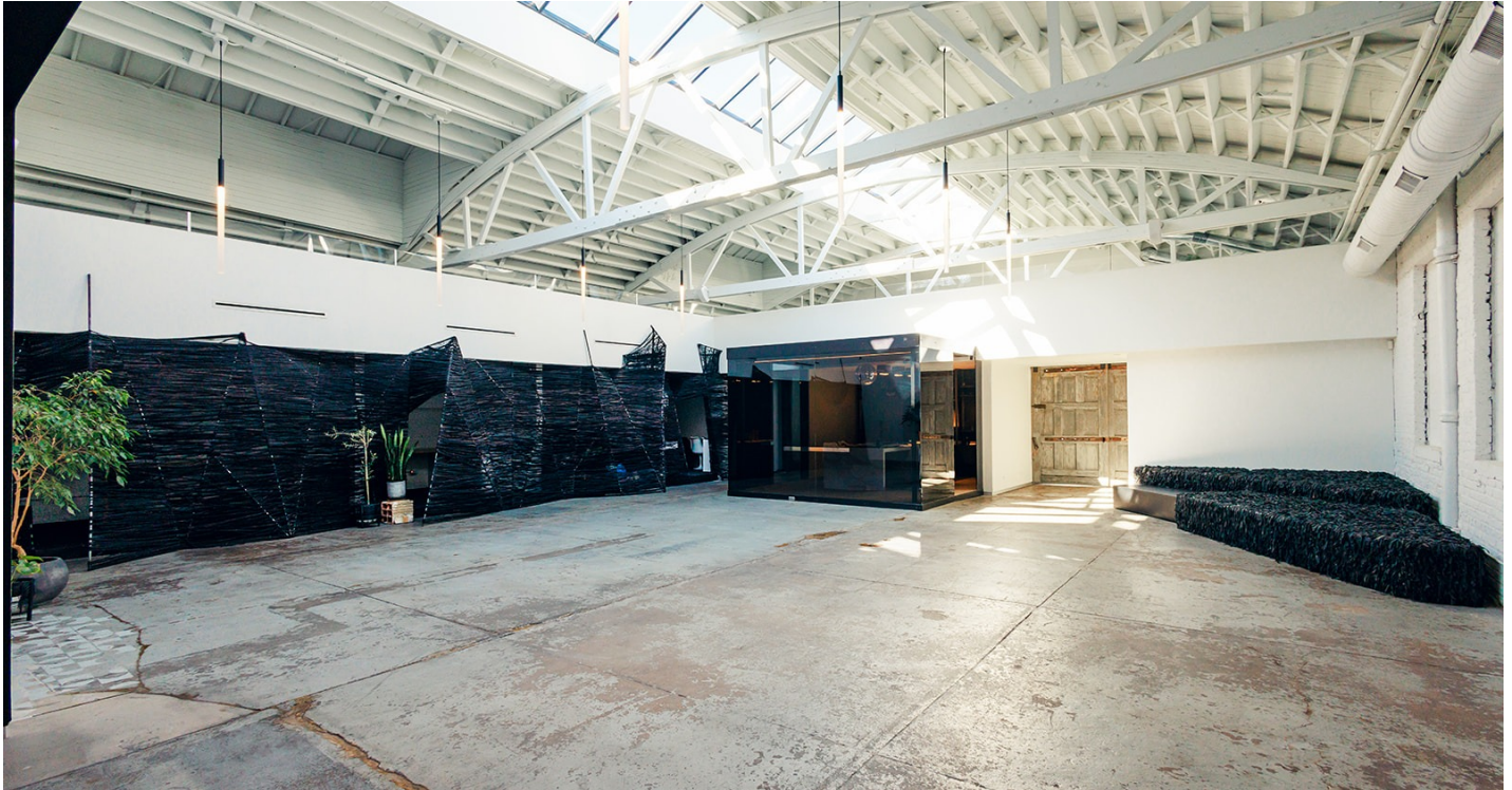
INTERIOR Clear-span bow-truss structure with 75' operable skylight
