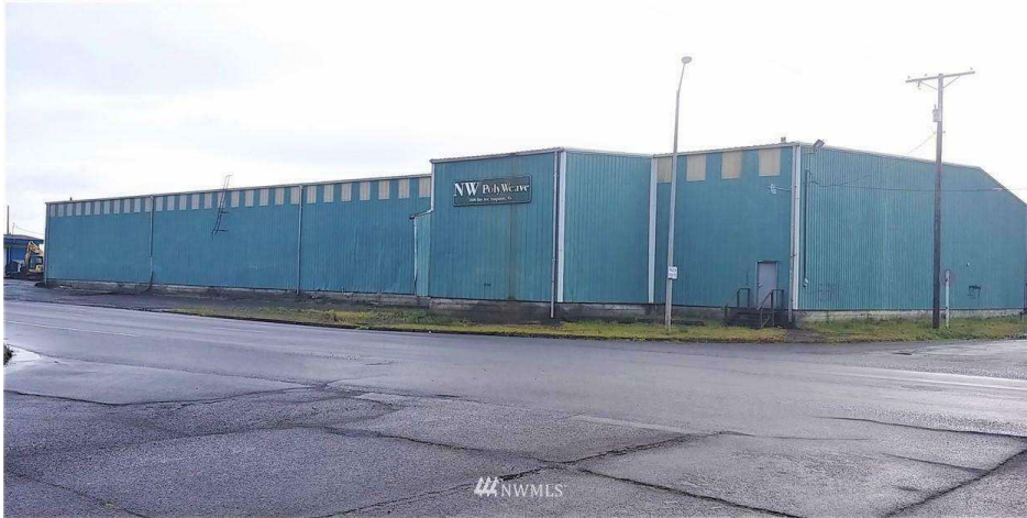
★ Grays Harbor Industrial Building 2600 Bay Ave, Hoquiam, WA 98550
