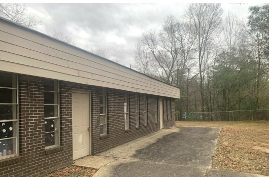
Building- Right Side
