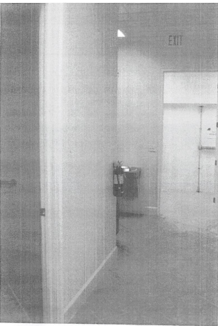
⑪ REAR HALLWAY - SOUTH
