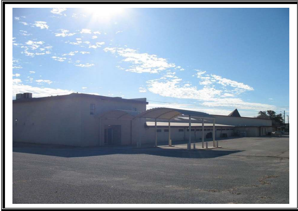
Southeasterly view of subject property, February 1, 2024.
