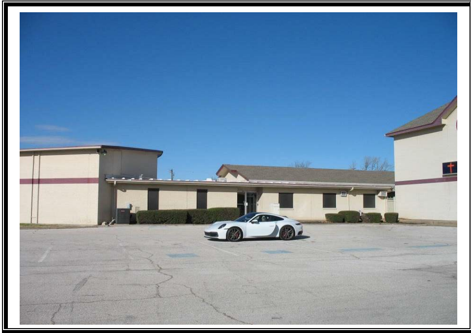
Westerly view of subject property, February 1, 2024.
