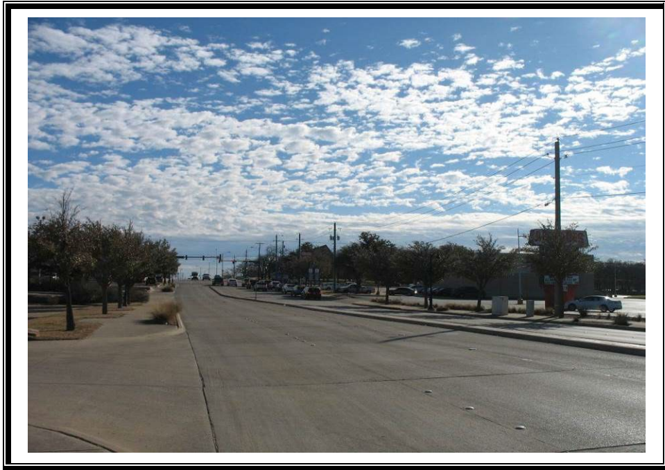
Easterly view of W. Pipeline Road, February 1, 2024.
