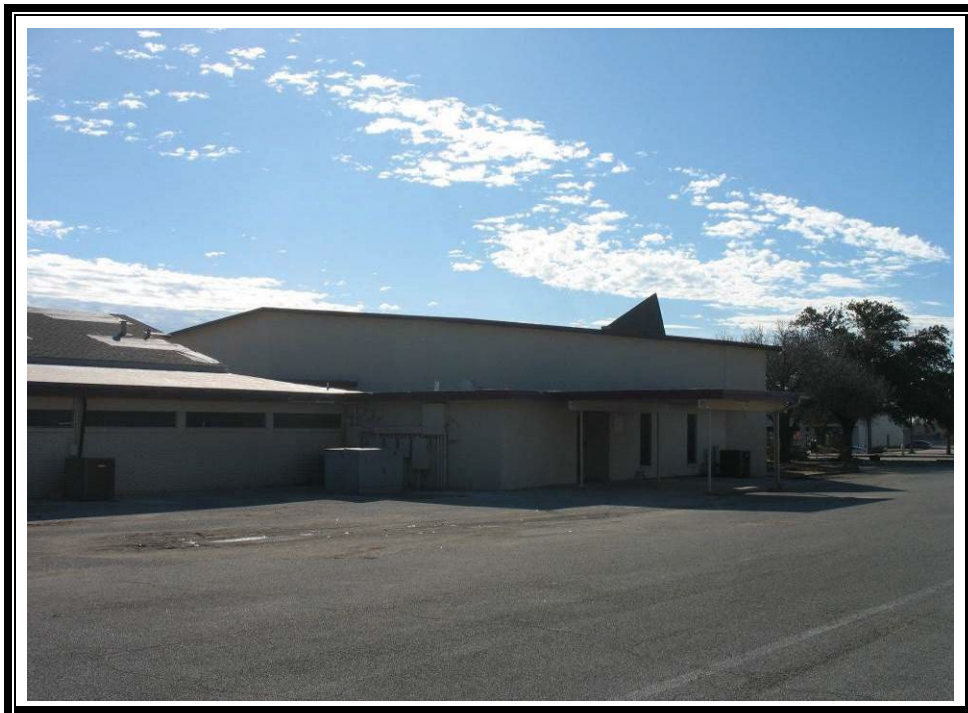
Southeasterly view of subject property, February 1, 2024.
