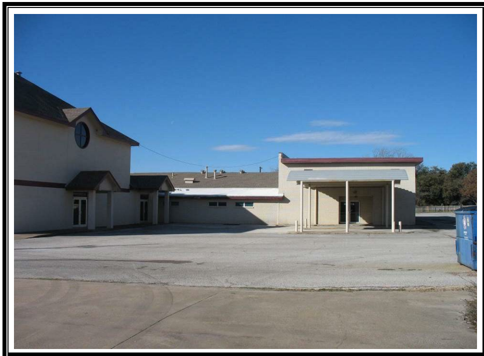
Westerly view of subject property, February 1, 2024.
