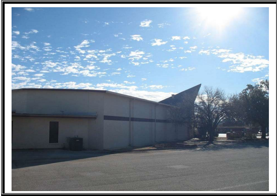
Southeasterly view of subject property, February 1, 2024.
