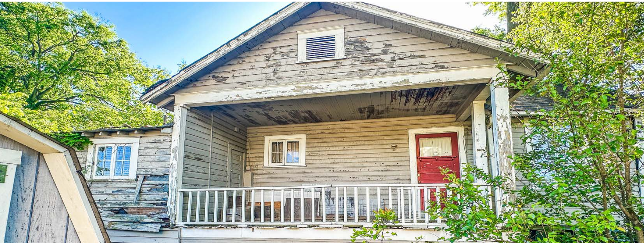
EXTERIOR PHOTOS (REAR STRUCTURE)
