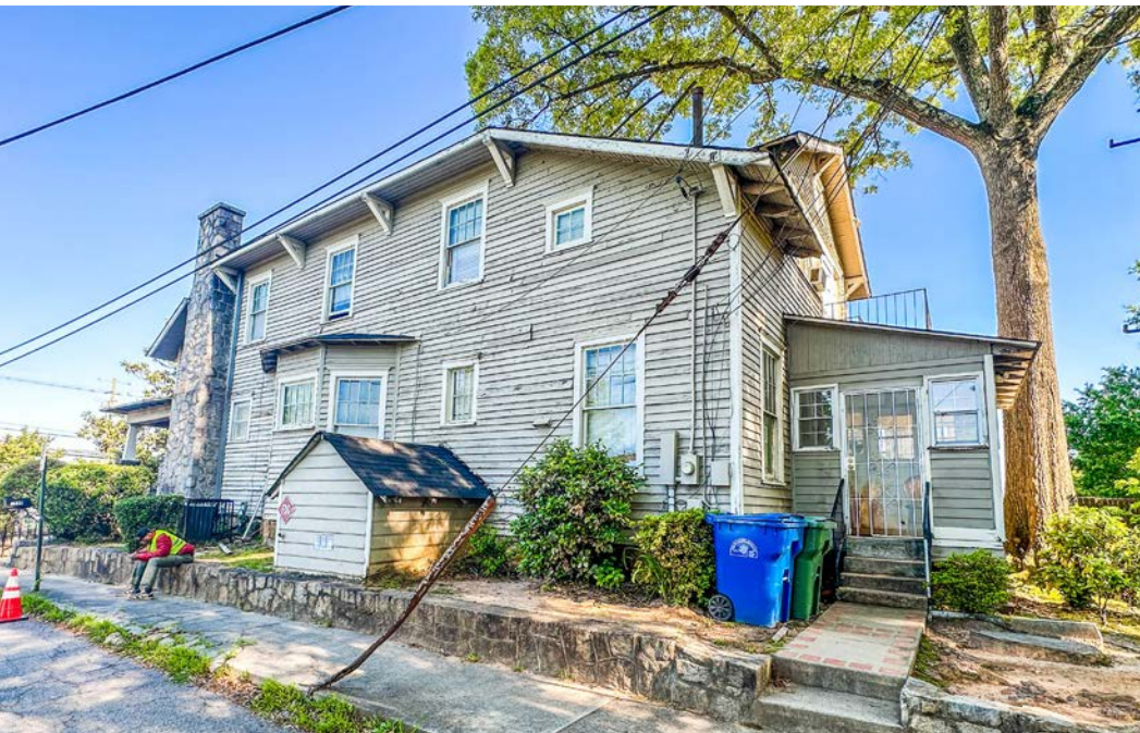
EXTERIOR PHOTOS (MAIN STRUCTURE)
