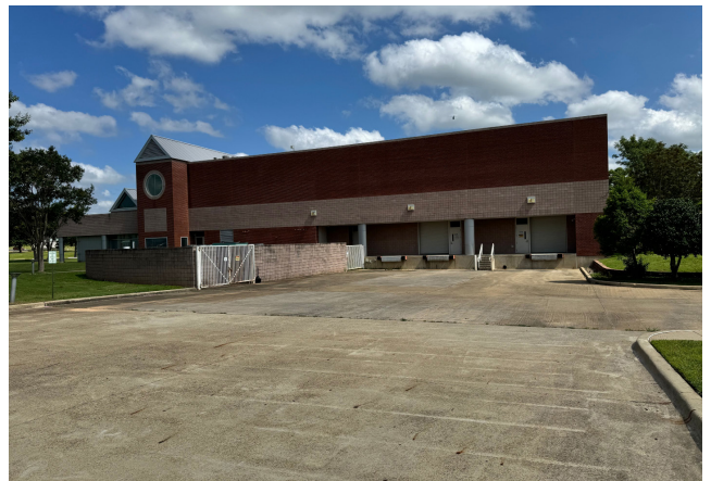
South Side - Dock Area
