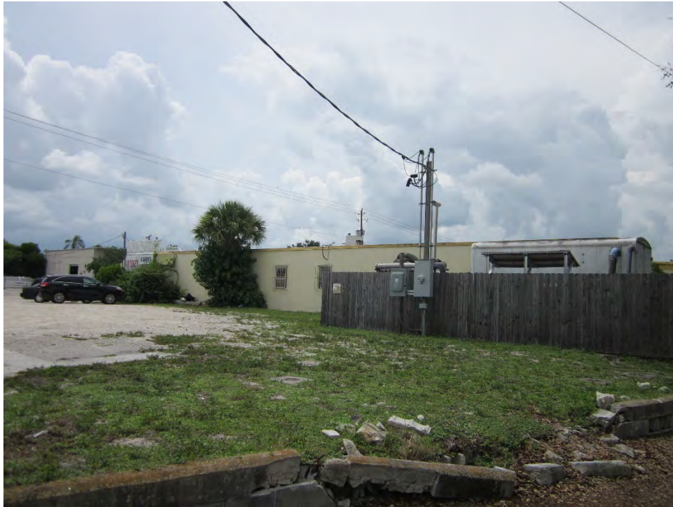
Site Photograph 45 – Remediation system located west adjacent to the southern portion of the Property
