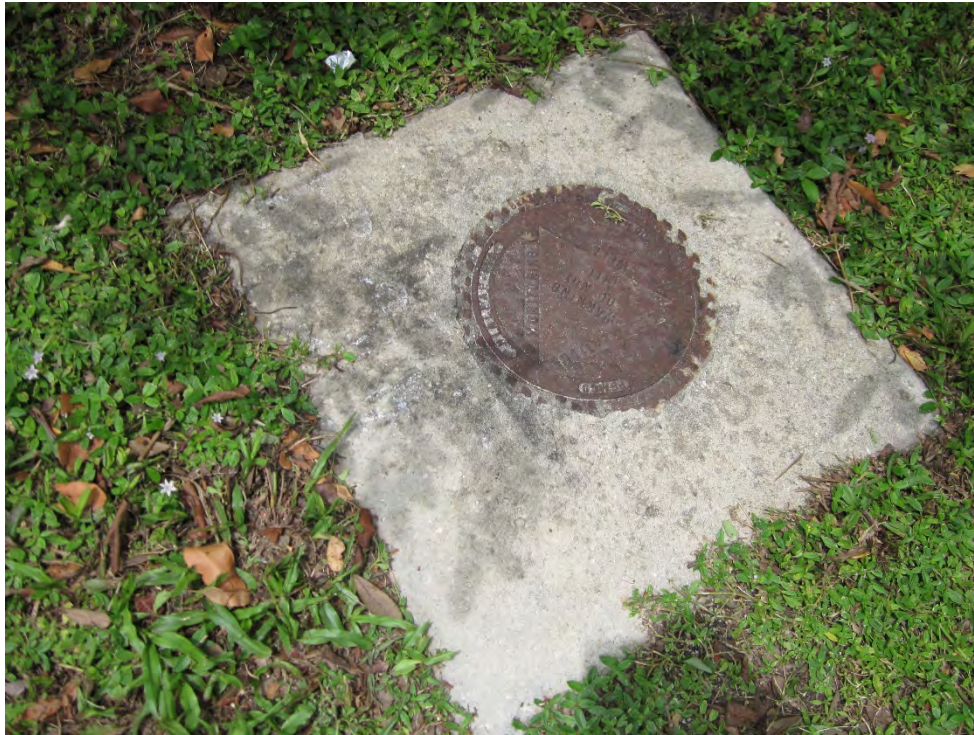
Site Photograph 37 – Representative photo of monitoring wells scattered throughout the Property
