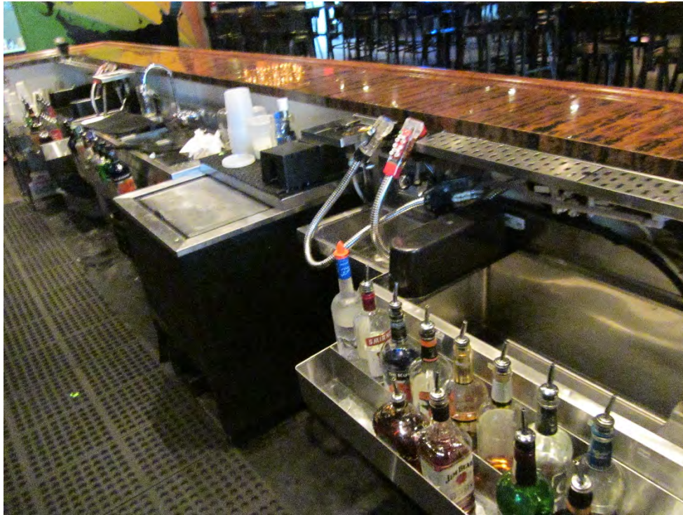
Site Photograph 11 – Area located behind the bar of FFCB
