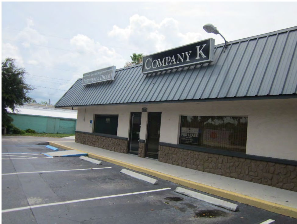
Site Photograph 26 – West side of south Property building (currently vacant)
