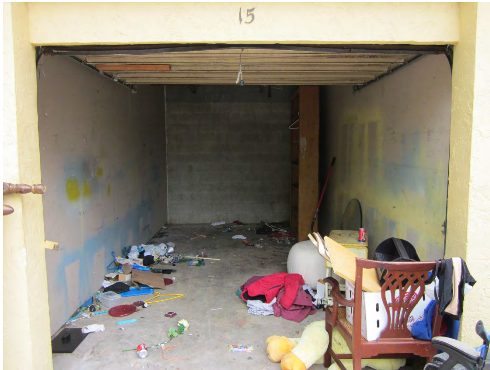
Site Photograph 33 – Representative photo inside storage unit
