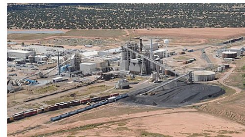
Novo Biopower Plant
