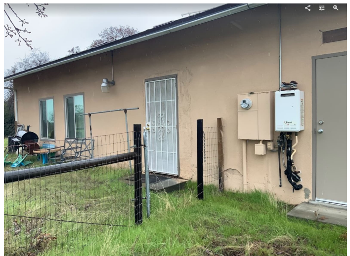
Rear of Church building
