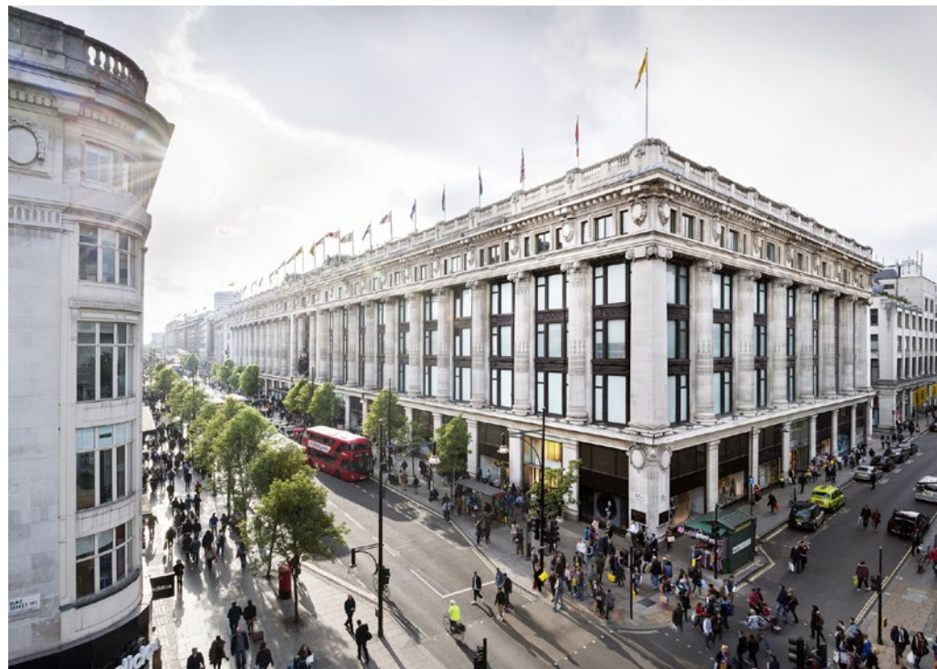
ONE OF THE MANY CENTRAL PERKS OF 14 CAVENDISH SQUARE
