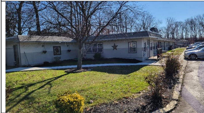
Viewing the subject exterior from the entrance from Corkery Lane.
