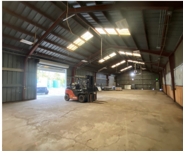
WAREHOUSE A INTERIOR:
