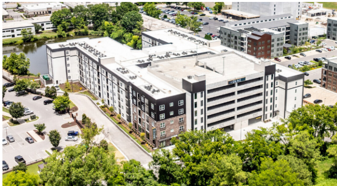
THE DUKE AT METROCENTER 194 UNITS (2024)
