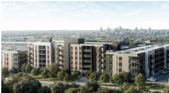
NORTHVIEW 254 UNITS (UNDER CONSTRUCTION)
