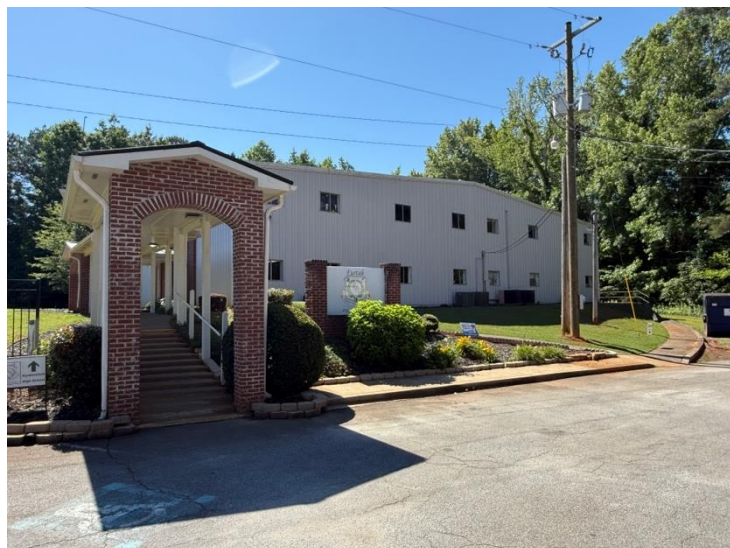
Gym and Classroom Building
