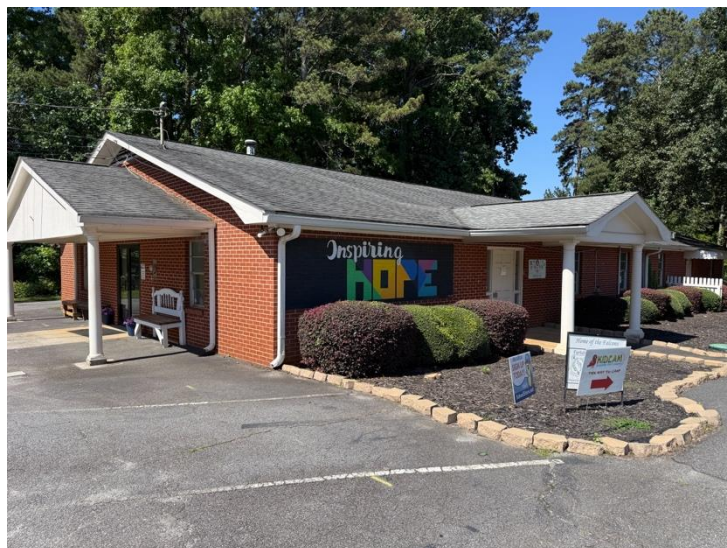
Activity Building with Large Rooms
