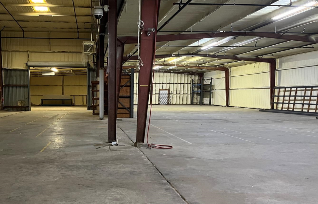
Entire Bay Space
