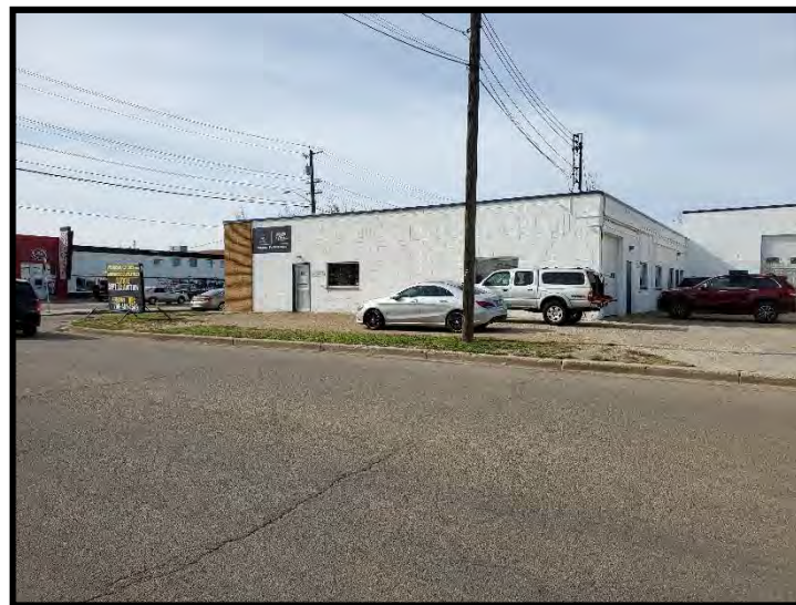
Photo 8 – Photograph of the subject site facing south west.
