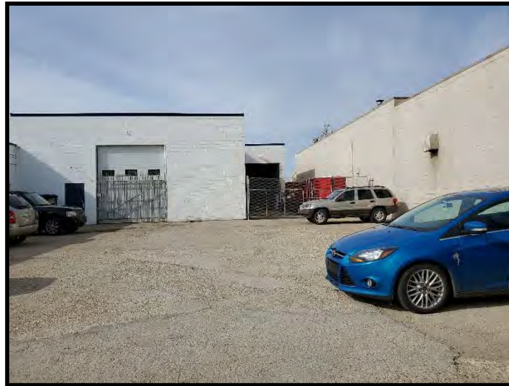
Photo 11 – Photograph of the parking lot and loading bays facing west.
