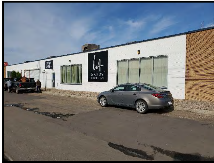
Photo 1 – Photograph of the subject site building and entrance facing north west.
