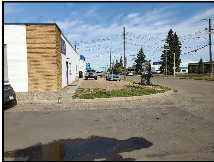
Photo 2 – Photograph of the subject site building, parking lot and parking lot entrance facing north.
