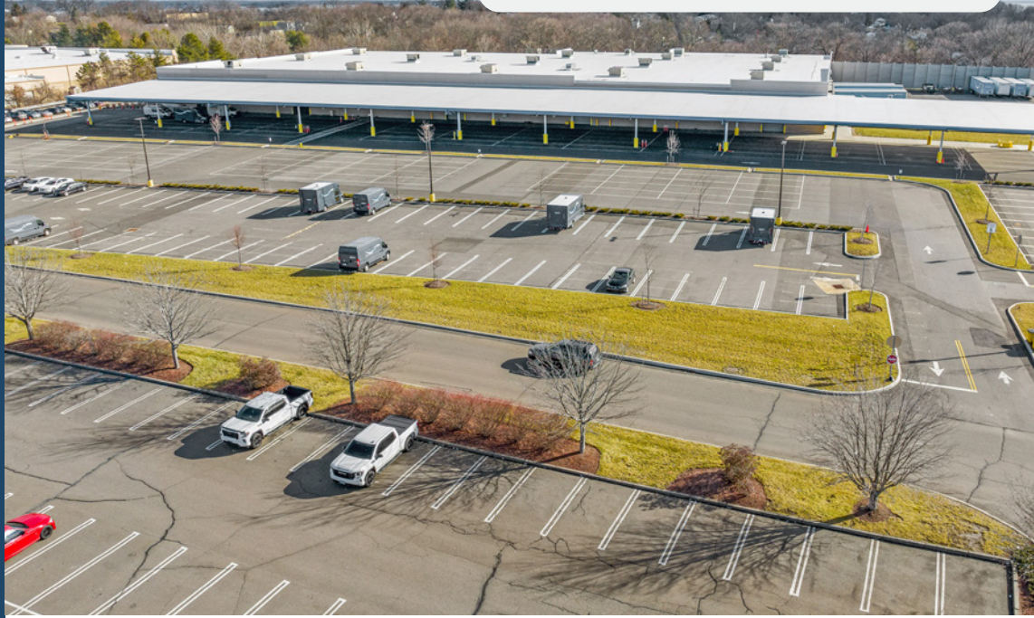
Amazon Distribution Center
