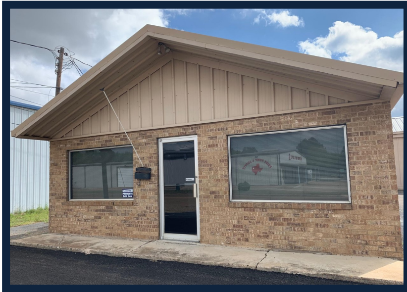
Front Entry to Office Area
