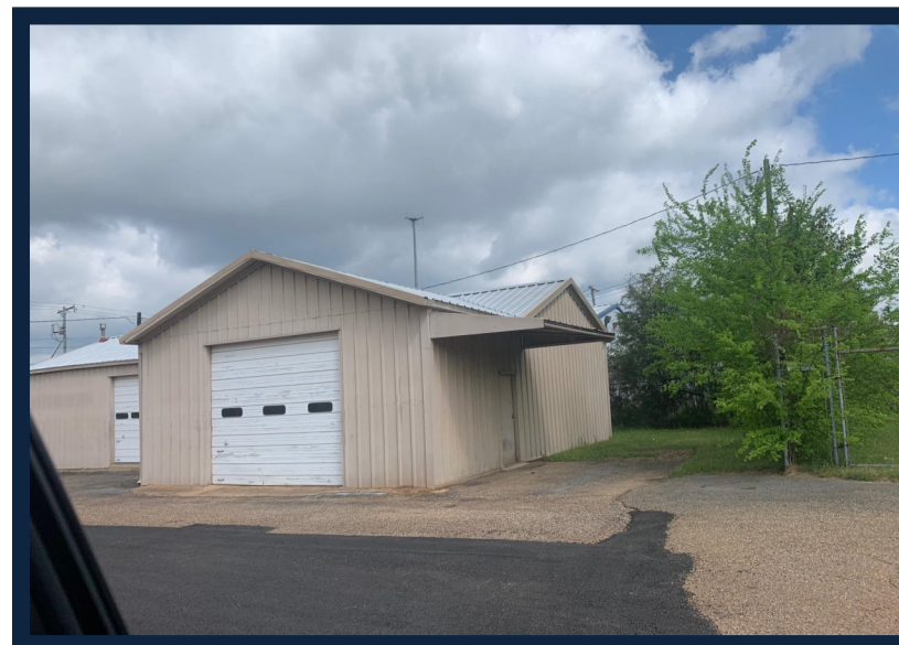
Rear Canopy Area Behind Building for Some Outside Storage
