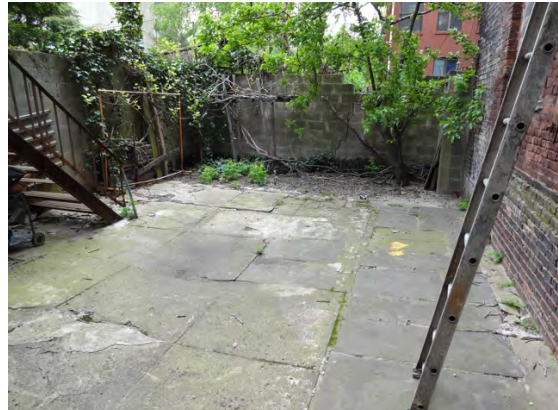
REAR YARD FROM 1 ST FLOOR
