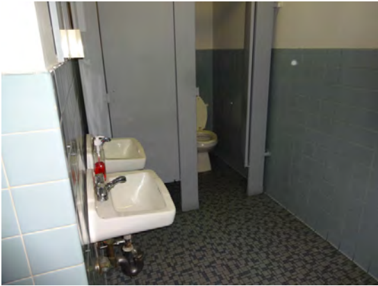
MEZZANINE LEVEL LAVATORY #1
