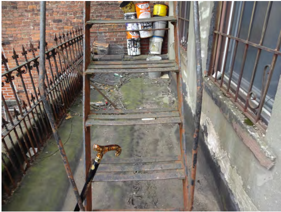
2 ND FLOOR REAR TERRACE
