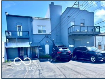
Back Of Structure
