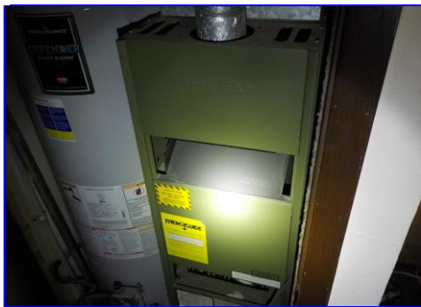
Unit 3 heater is old and is the 65% style.
