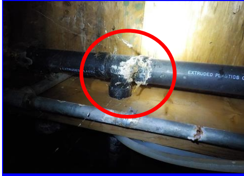
The kitchen drain under unit 7 is broken and leaking as seen from the crawl space.
