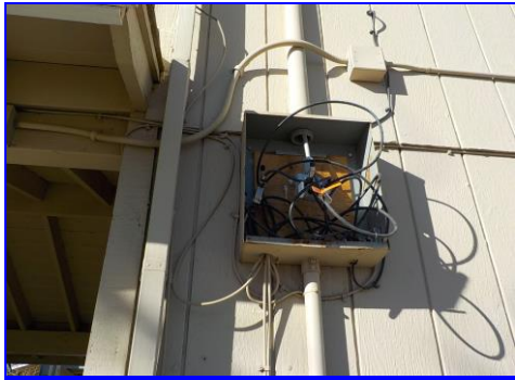
The cover to the cable TV on the east building is off.
