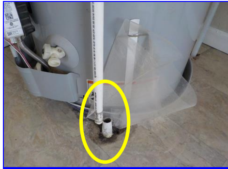
The laundry water heater relief valve pipe is out of place and is leaking.
