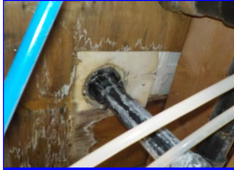
The shower drain in the studio apartment is leaking as seen from the crawl space.
