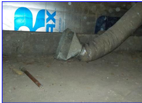
One duct under unit 2 has fallen off.
