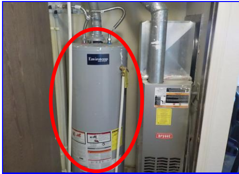
The water heaters are missing the approved seismic straps.
