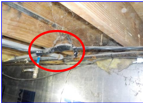
There is a wire splice under the studio apartment that is not in a junction box.
