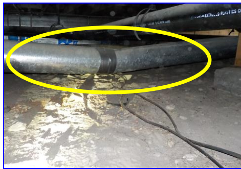
One duct under unit one is missing a strap and the pipe is bending at the joint.
