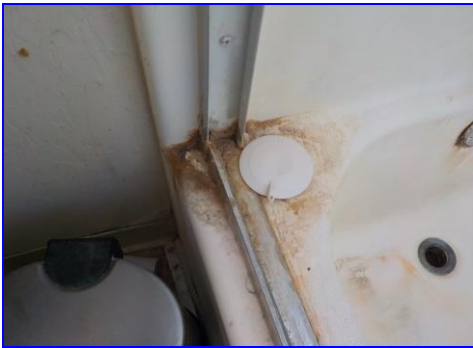
The tub/shower door is leaking at the corner. Clean and re-seal. Unit 7.
