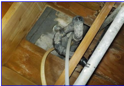
Unit 2 has a leak under the tub.
