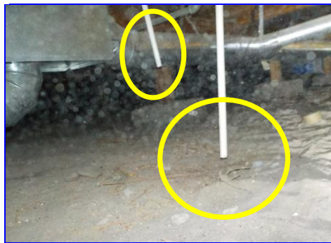
Water heater relief valve piping should be extended to the exterior with no up turns.
