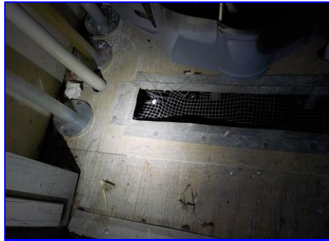
The heater combustion air vent in the floor is damaged in unit 1.
