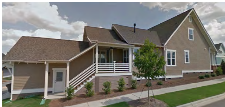
This house has multiple windows, a side porch, and varying levels of stories.
