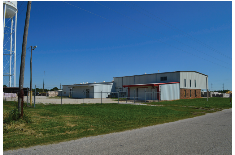
Property Looking East
