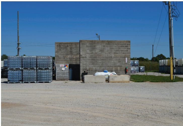
12" Concrete Block Containment Area
