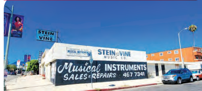
Gregory Avenue frontage
