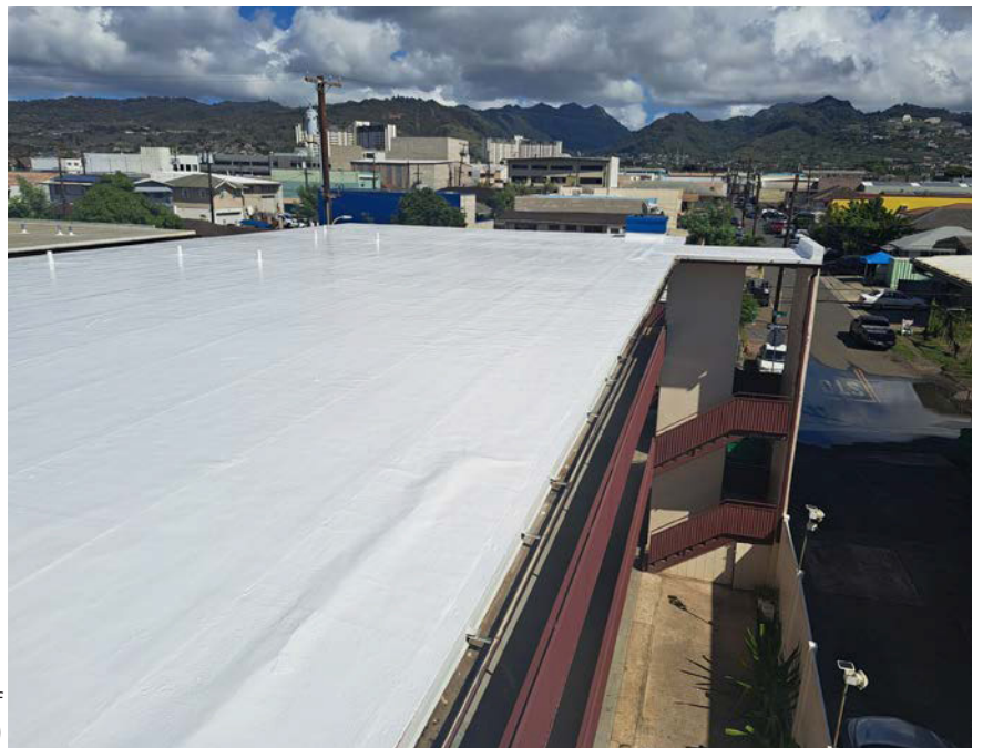
New Roof (Nov. 2022)
