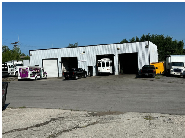
4,000 SF building with D.I. doors
