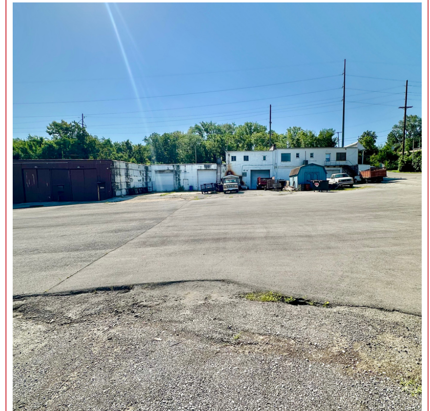
Back of Manchester Trfy Frontage Building
