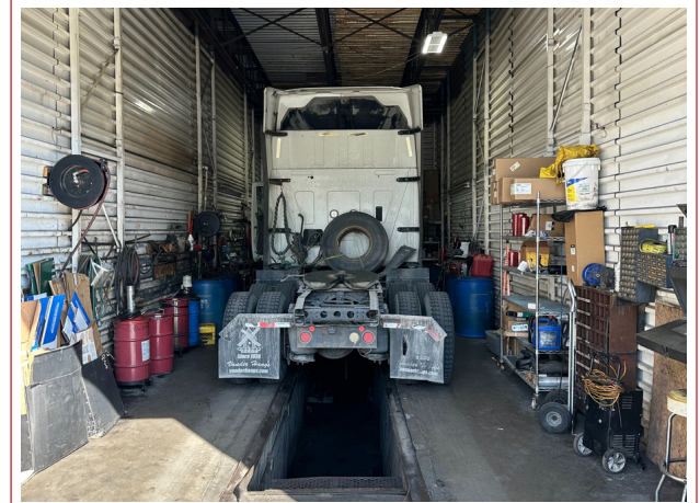
Truck bay with maintenance pit
