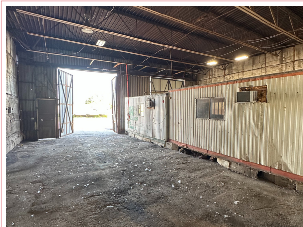
6,000 SF building interior
