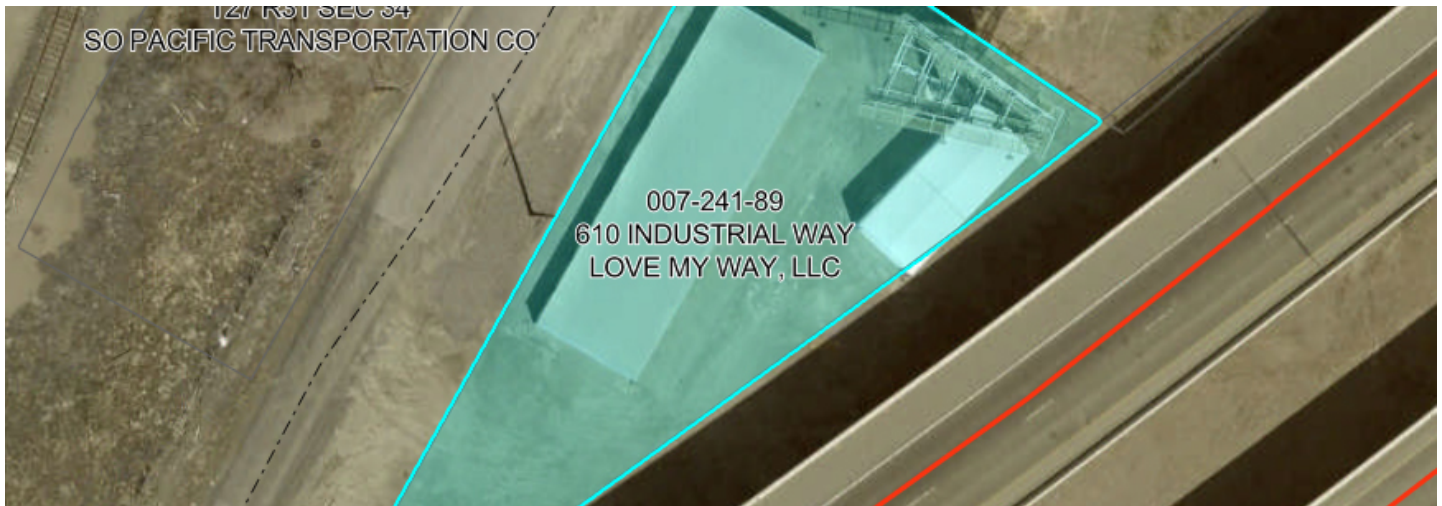
Aerial view showing property boundaries and layout of 610 Industrial Way
