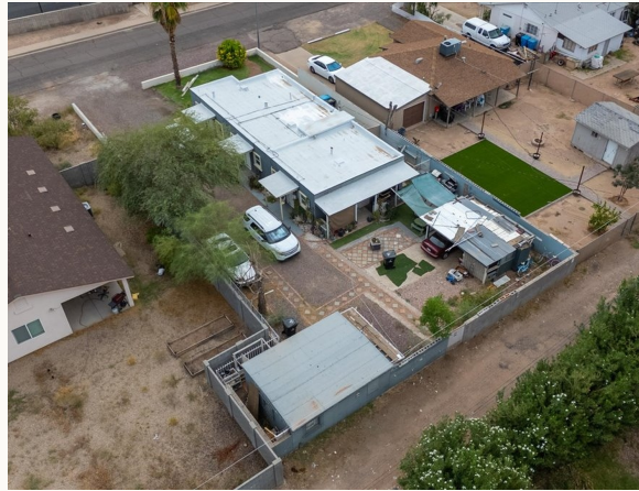
AERIAL — SITE AND PARKING
