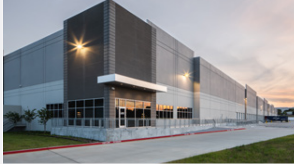
// PARC SOUTHWEST IRVING, TEXAS
