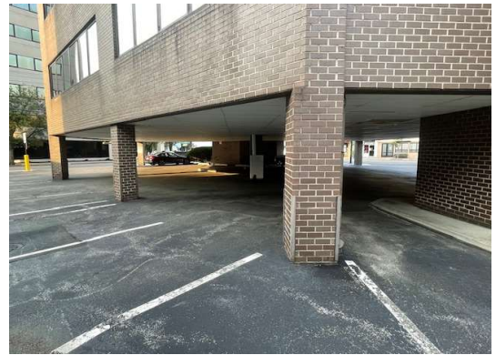
On-Site, Covered Parking
