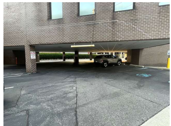
On-Site, Covered Parking
