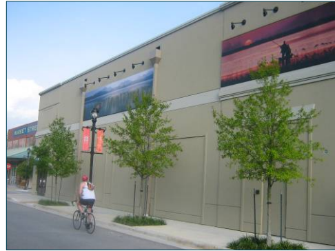
Every side of the building façade should incorporate architectural elements to eliminate the appearance of blank walls.
