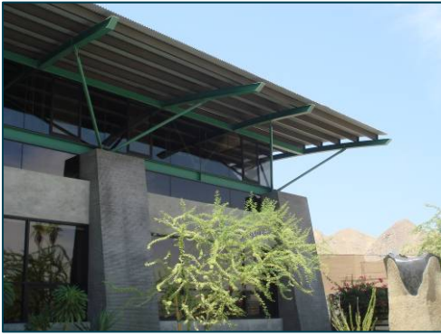
Solar orientation of the building, overhangs, and other devices placed on the exterior of buildings reduce direct sunlight into interiors, lowering heat gain and the amount of energy needed for cooling.
