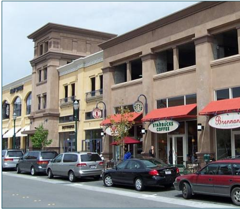
Example of a mixed-use structure with parking incorporated on the upper levels.
