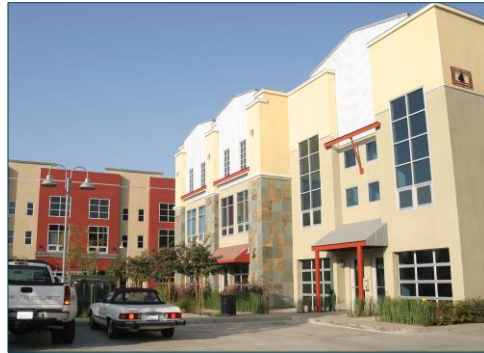
Example of live/work units, with office space on the ground floor and residential space above.
