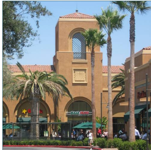
Tower features add a landmark character to the project.
