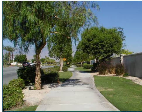
The 8-foot-wide sidewalk accommodates pedestrians, cyclists, and golf carts.
