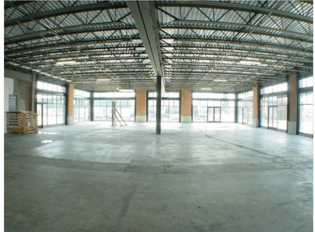
Heavy Gauge Exposed Steel Interior with Rooftop Insulation
