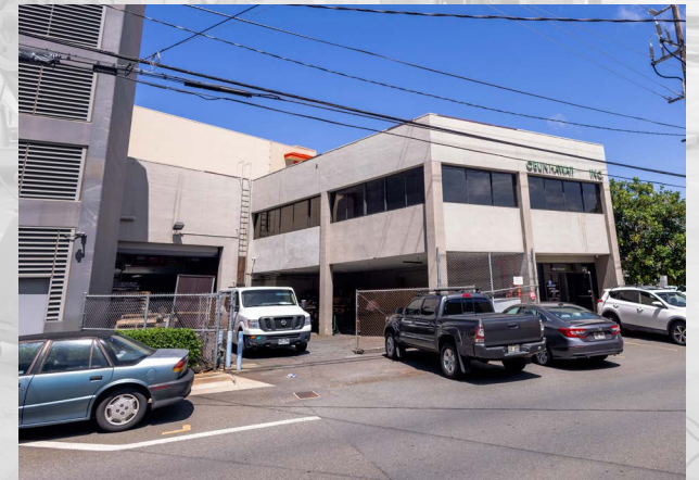
Yard and parking fronting the building
