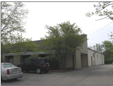
Front of Building
